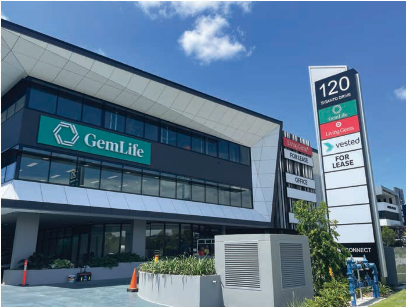
GEMLIFE'S NEW NATIONAL HEADQUARTERS AT HELENSVALE, QUEENSLAND
