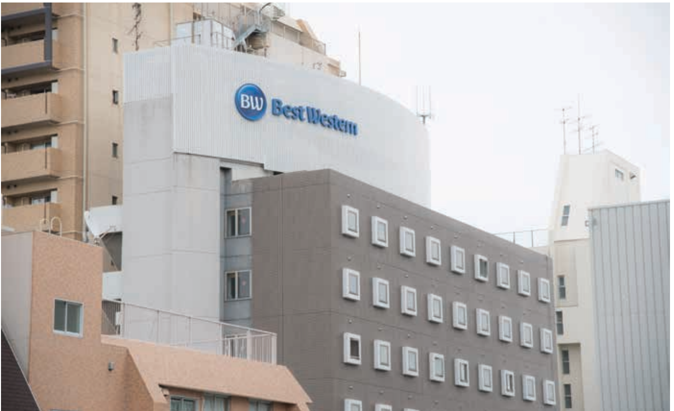
BEST WESTERN OSAKA TSUKAMOTO HOTEL, TSUKAMOTO • LAND AREA - 525 SQM • EFFECTIVE OWNERSHIP - 50% • NO. OF ROOMS - 105
