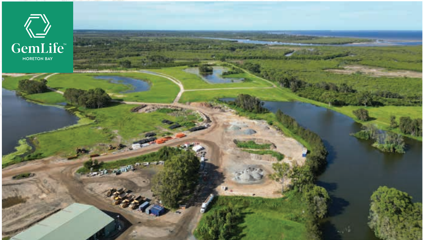
STAGE ONE LAUNCHED IN Q4 2023 AND HOUSE CONSTRUCTION COMMENCED IN Q1 2024
