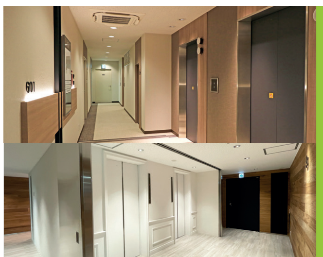
Renovation works including change of elevator and energy efficient air-cons & LED lighting
