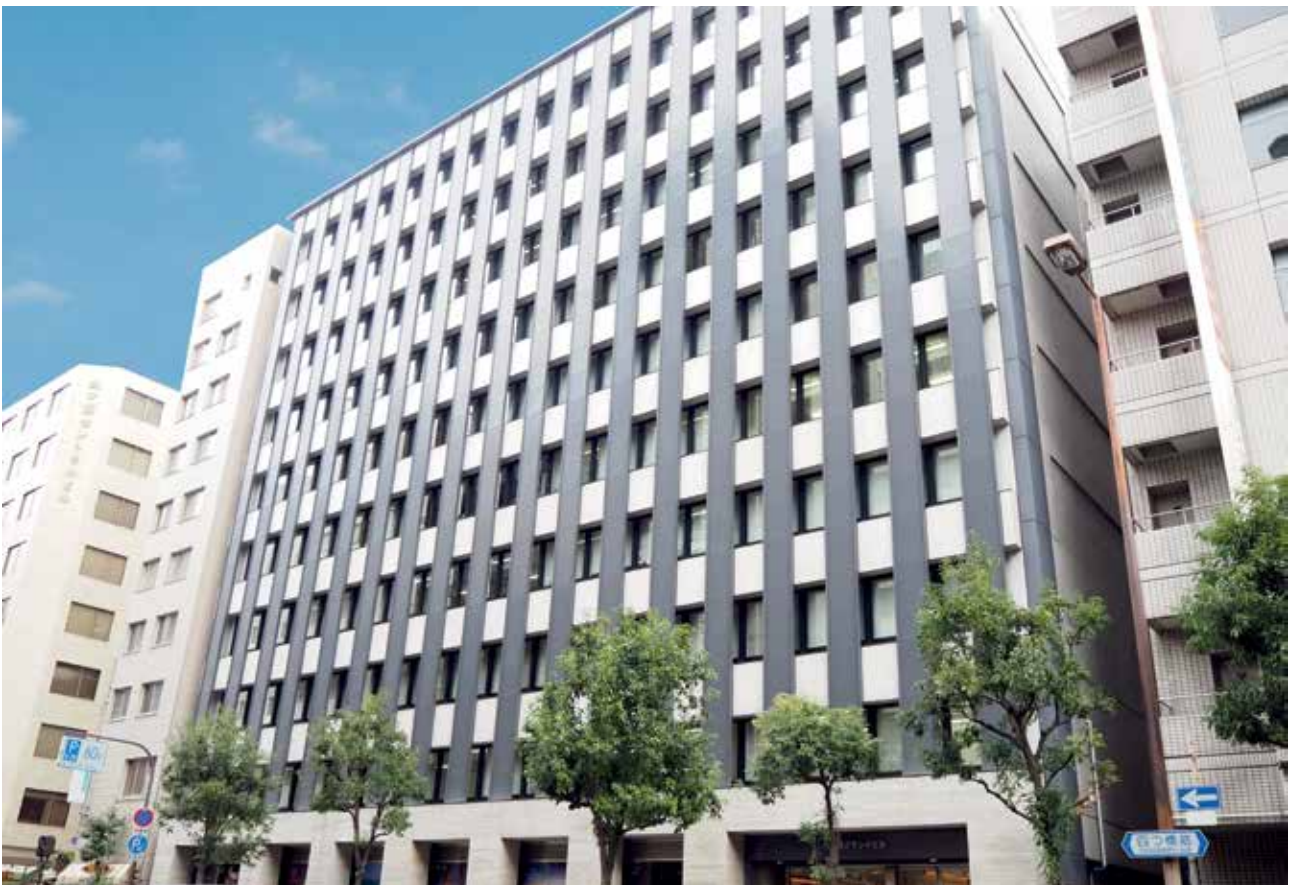
YOTSUBASHI GRAND BUILDING, BROAD STREET FRONTAGE ON YOTSUBASHI SUJI, SHINSAIBASHI • LAND AREA - 881 SQM • GFA - 7,524 SQM • EFFECTIVE OWNERSHIP - 55%
