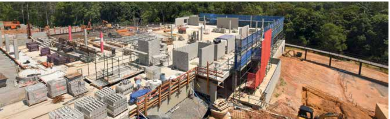
CONSTRUCTION FOR COUNTRY CLUB COMMENCED IN FEBRUARY 2023
