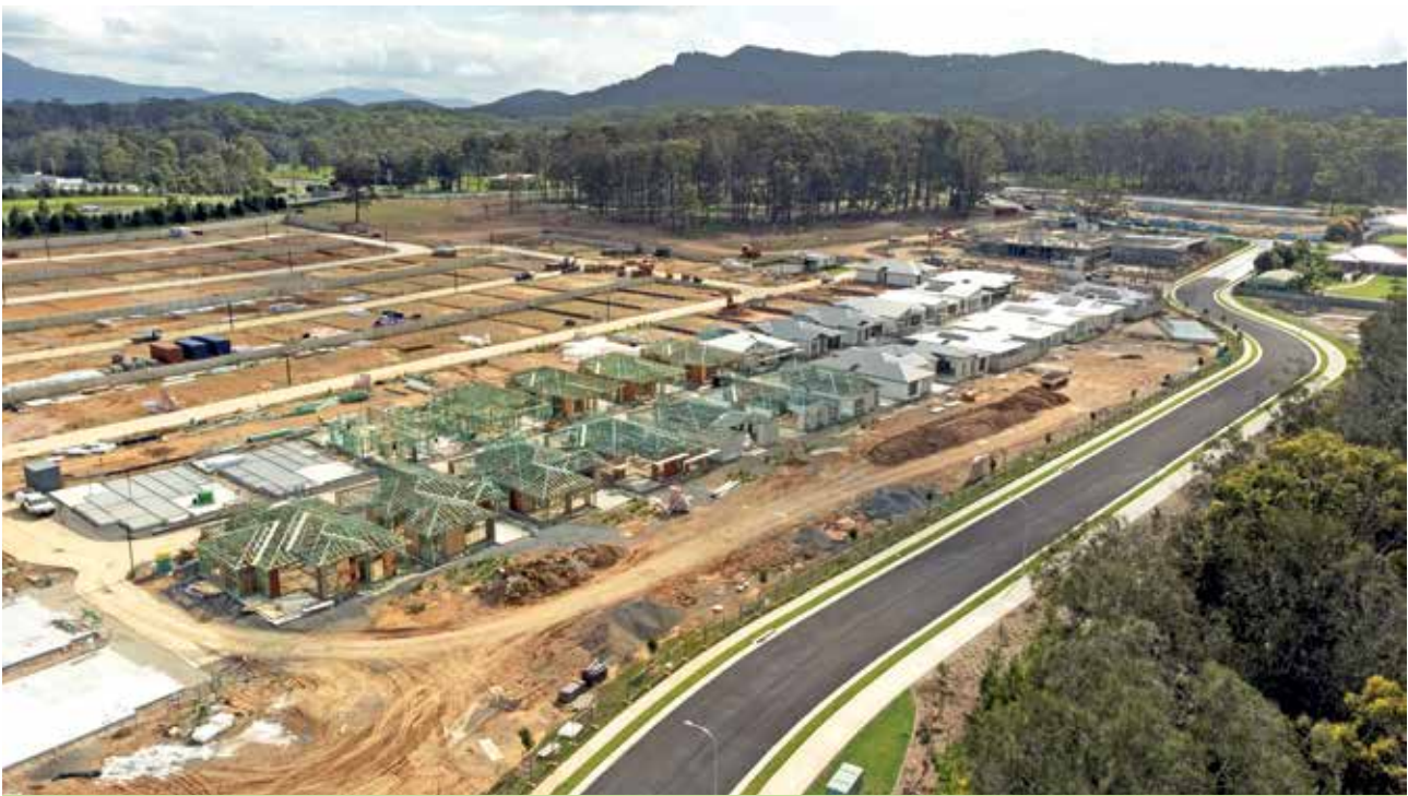
CIVIL WORKS ACROSS THE SITE COMPLETED IN DECEMBER 2022
