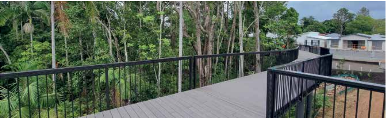
313 METRES OF ELEVATED BOARDWALK TAKING SHAPE
