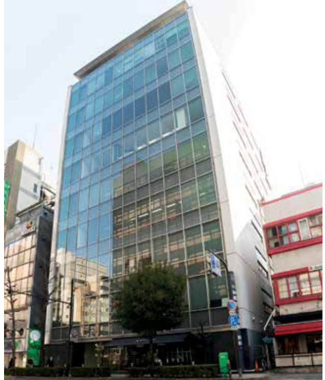
YOTSUBASHI NAKANO BUILDING ALONG YOTSUBASHI SUJI, SHINSAIBASHI • LAND AREA - 806 SQM • GFA - 7,925 SQM • EFFECTIVE OWNERSHIP - 50%
