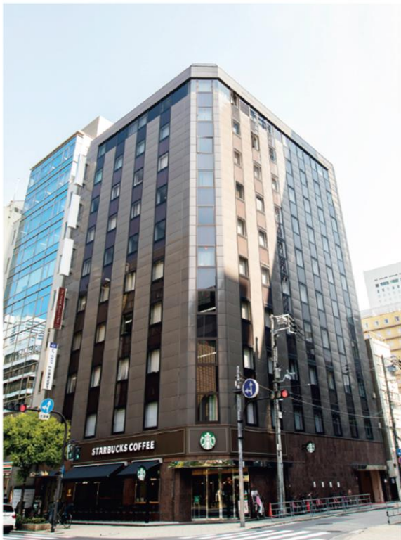
YOTSUBASHI EAST BUILDING AT THE CORNER OF YOTUSBASHI SUJI, SHINSAIBASHI • LAND AREA - 525 SQM • GFA - 4,695 SQM • EFFECTIVE OWNERSHIP - 50%
