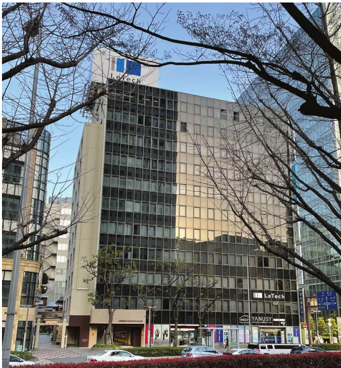
UMEDA PACIFIC BUILDING
