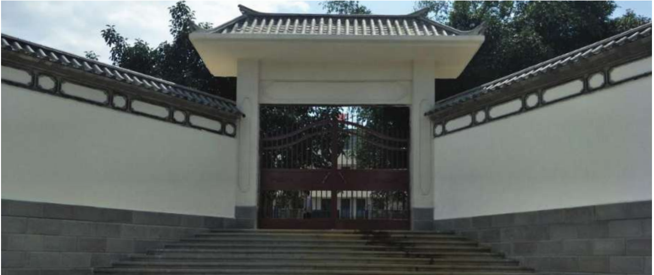
Figure 19: Restoration and construction works for Manhattan Primary School:
