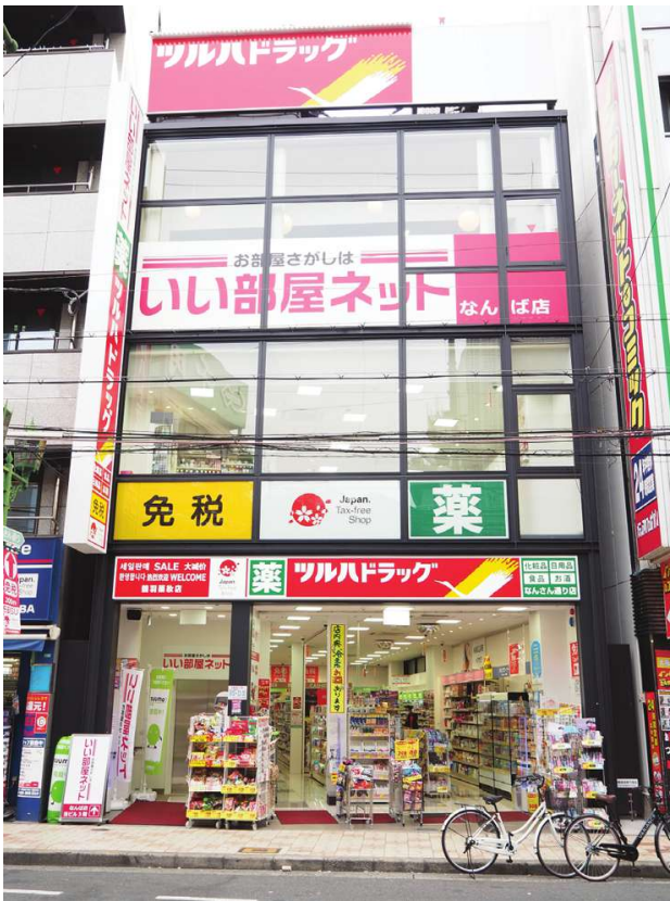
NAMBANAKA THAKRAL BUILDING
