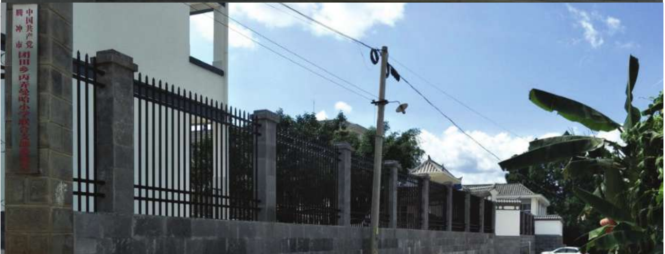
SCHOOL GATE, BLUESTONE STEPS AND GUARDRAIL CONSTRUCTED
