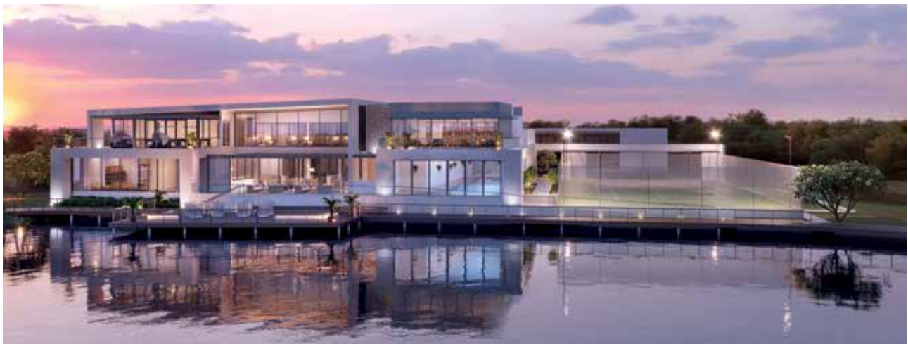
CONSTRUCTION OF LAKESIDE COUNTRY CLUB WELL UNDERWAY
