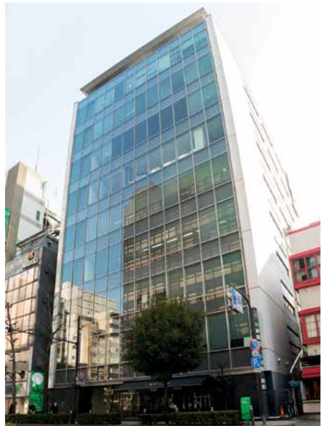
YOTSUBASHI NAKANO BUILDING ON YOTUSBASHI SUJI, SHINSAIBASHI • LAND AREA - 806 SQM • GFA - 7,925 SQM • EFFECTIVE OWNERSHIP - 50%
