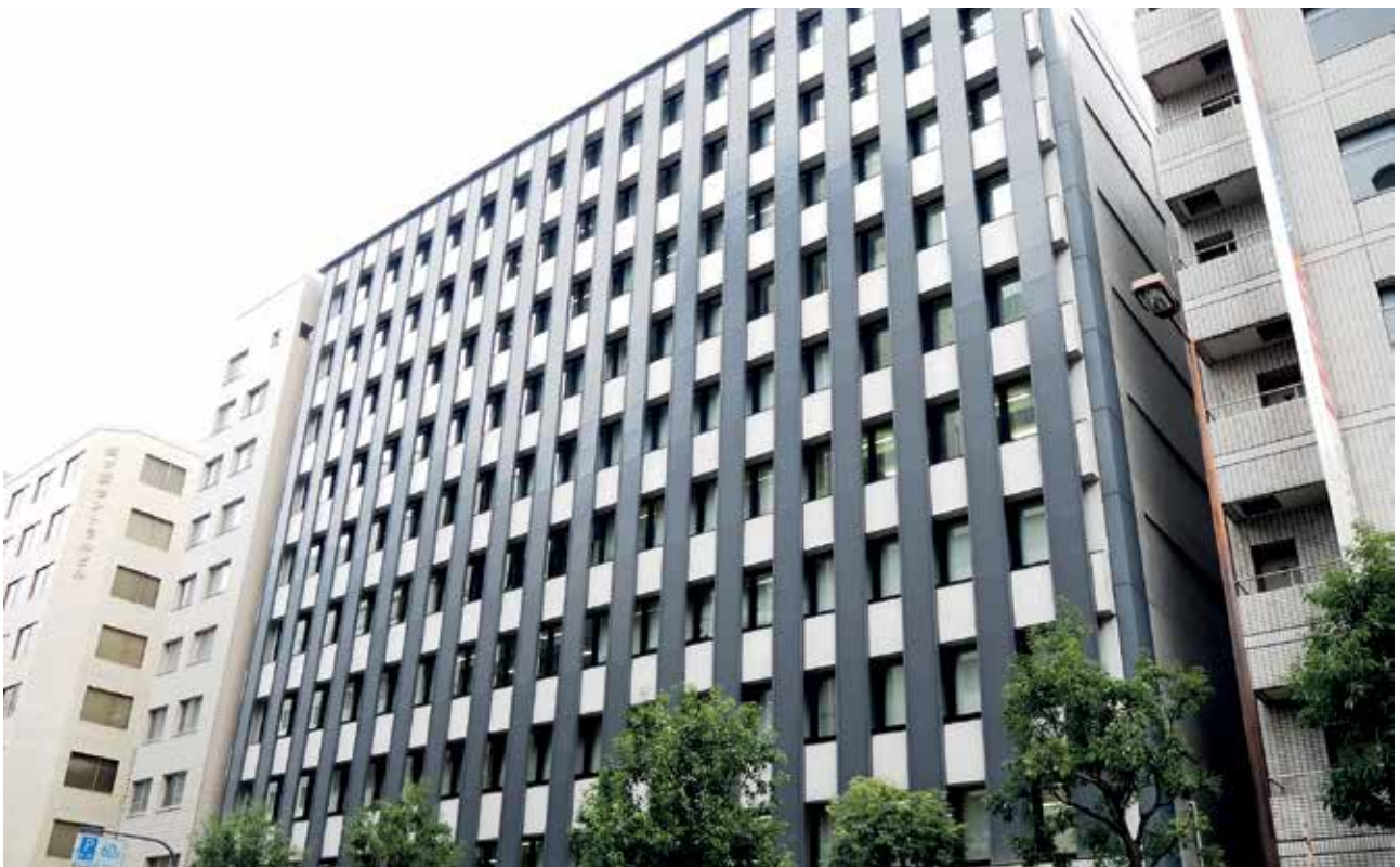
YOTSUBASHI GRAND BUILDING, BROAD STREET FRONTAGE ON YOTSUBASHI SUJI, SHINSAIBASHI • LAND AREA - 881 SQM • GFA - 7,524 SQM • EFFECTIVE OWNERSHIP - 53%
