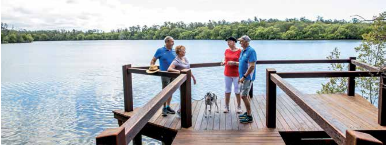
WORK ON THE 2-KM BOARDWALK MOVED INTO THE FINAL STAGES
