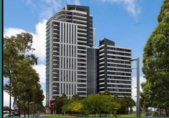
Australia Towers Stage 1 Sydney
