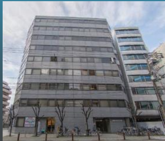
ITACHIBORI SQUARE BUILDING
