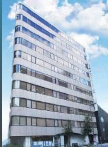
RIVERPOINT KITAHAMA BUILDING
