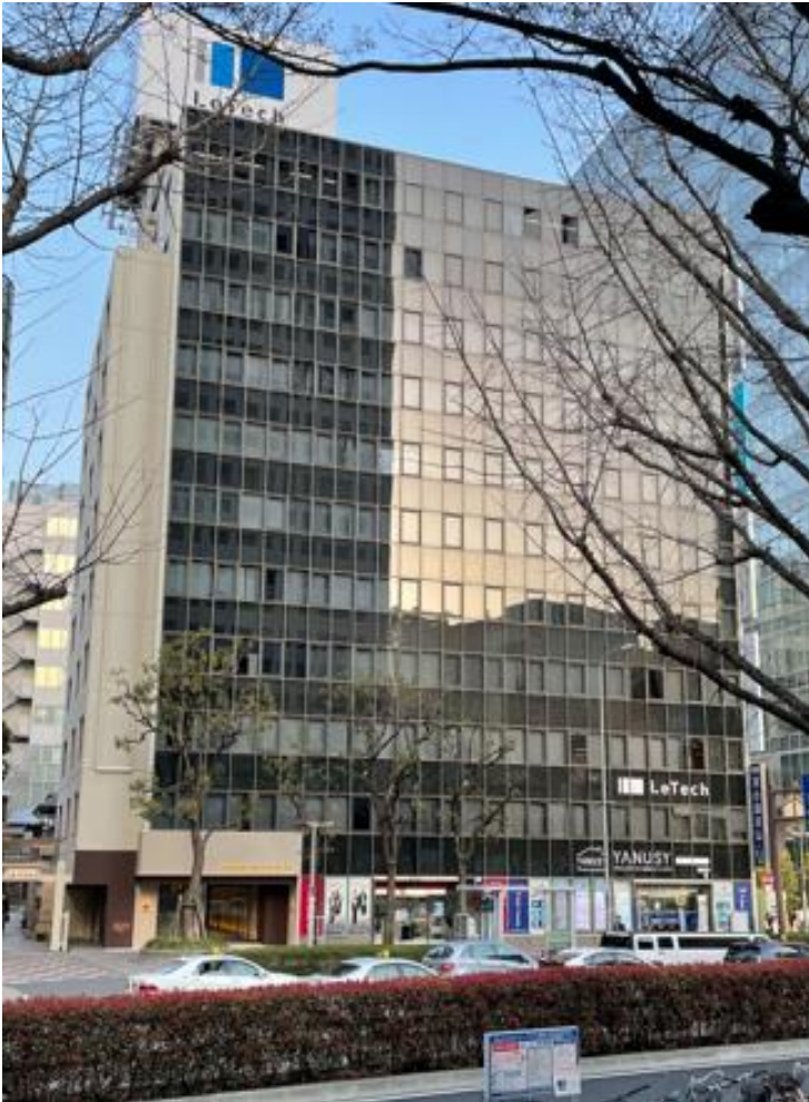
UMEDA PACIFIC BUILDING
