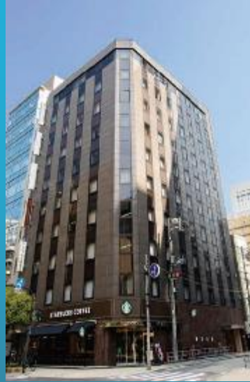
YOTSUBASHI EAST BUILDING
