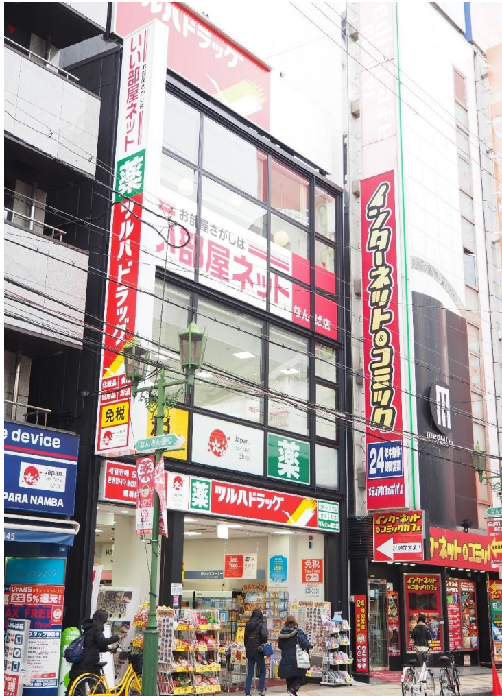
NAMBANAKA THAKRAL BUILDING
