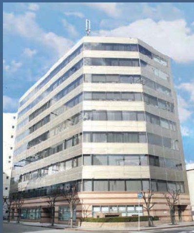
UTSUBO EAST BUILDING
