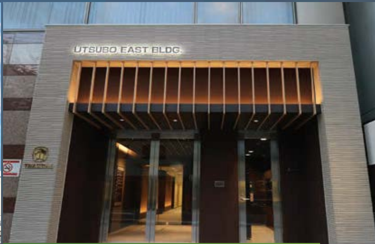
REFURBISHMENT OF UTSUBO EAST BUILDING
