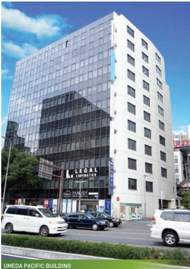
UMEDA PACIFIC BUILDING
